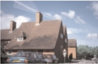
fig 5 Daneshill in 1999 as centrepiece of an office park
