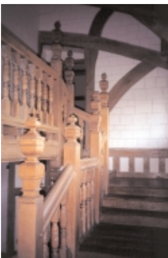
fig 2 The newel staircase at Deanery Garden after removal of the white paint
